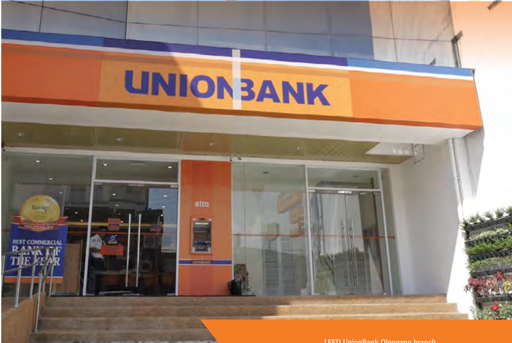
LEED UnionBank Olongapo branch
